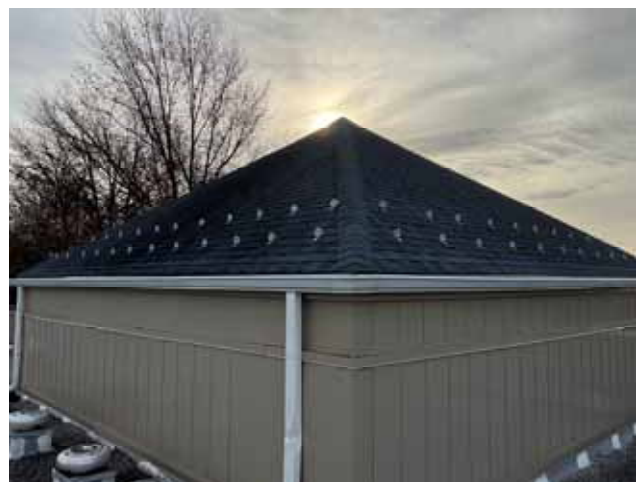
6 - SECONDARY ROOF OVERVIEW
