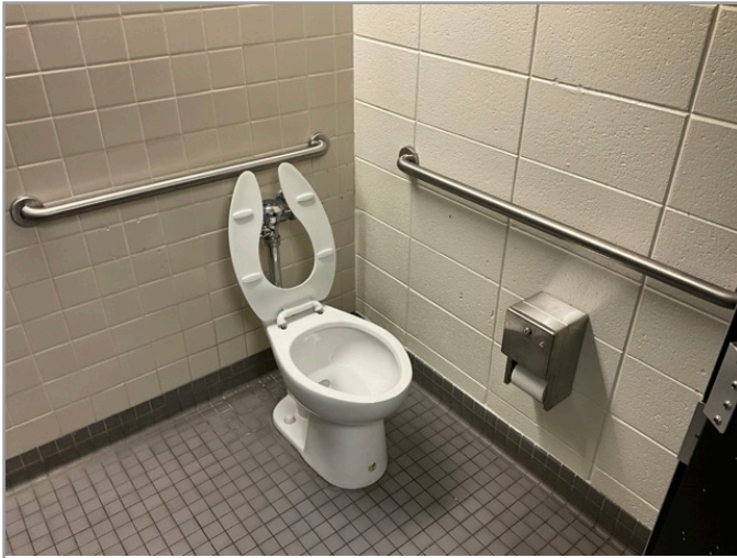
TOILET STALL OVERVIEW
