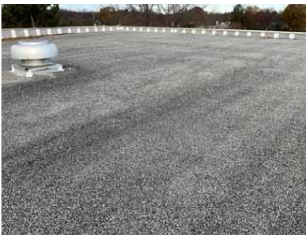
5 - PRIMARY ROOF OVERVIEW
