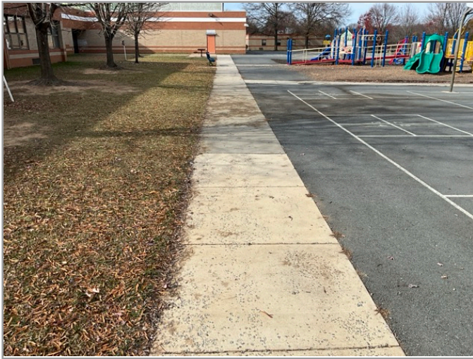
ACCESSIBLE ROUTE TO PLAYGROUND
