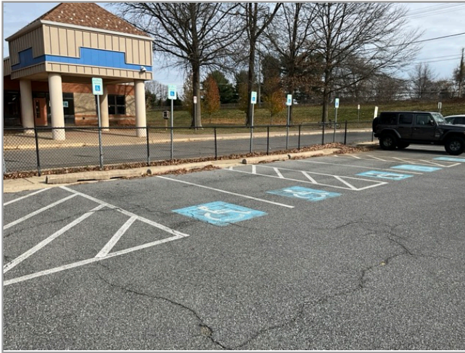
OVERVIEW OF ACCESSIBLE PARKING AREA
